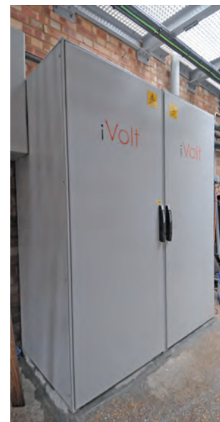
Outdoor IP cabinet for the iVolt installation
